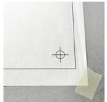
2. Use a drill to create one, 3/16" diameter hole through each of the four cross marks. Lightly hammer anchors into each of the four holes.
